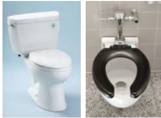
Tank-Type and Flushometer-Valve Toilets
